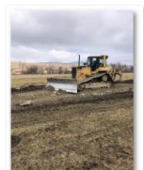
202102-Viaduct km 254+400 - Drum tehnologic_2
