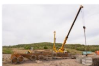
047_executie piloti portal P3 - tunel Homorod
