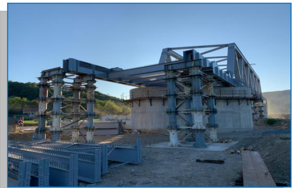
Premontare tablier metalic - Pod km 517+440
