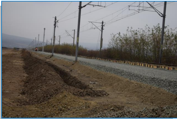
Terasament - Km 614 – Ghioroc
