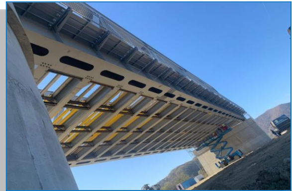
Cofrare tablier deschiderea - Pod km 517+440
