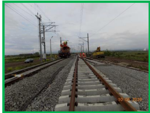
HM Podu Mures – Montare schimbator
