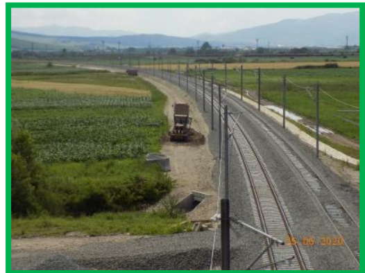
Km 396+300-396+550 Profilare drum tehnologic
