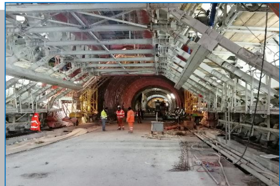
TUNEL - Front de cofrare
