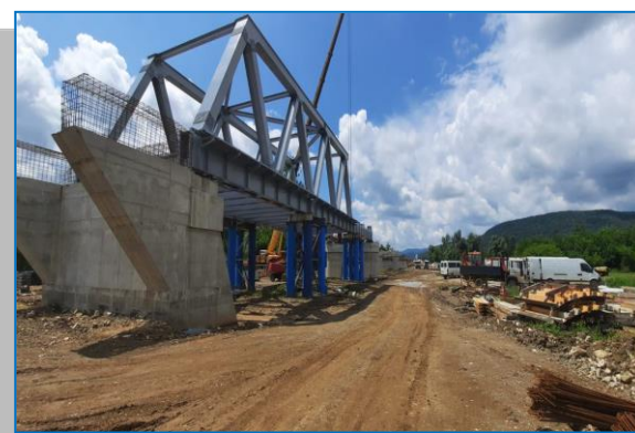
Montare tablier metalic – Pod km 517+440
