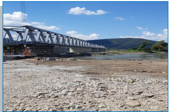
Montare tablier – Pod km 517+440
