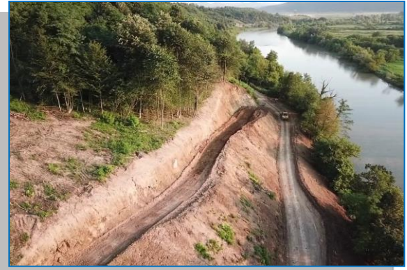
Realizare drum acces Tunel T1 – Iesire Polata km 523+757
