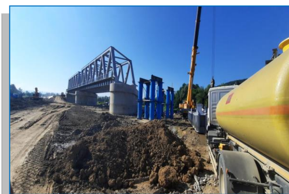
Montare tablier – Pod km 517+440
