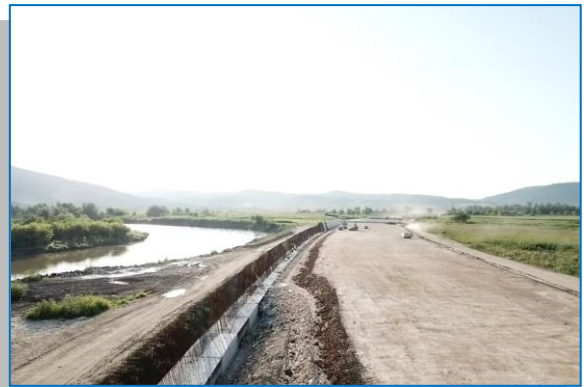
Executie zid de sprijin km 527+550- 527+650
