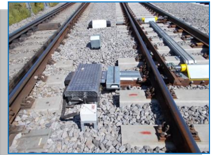
Blaj – electromecanism macaz
