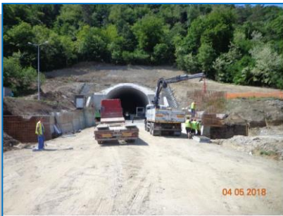
Armare camere de colectare Tunel Daneş
