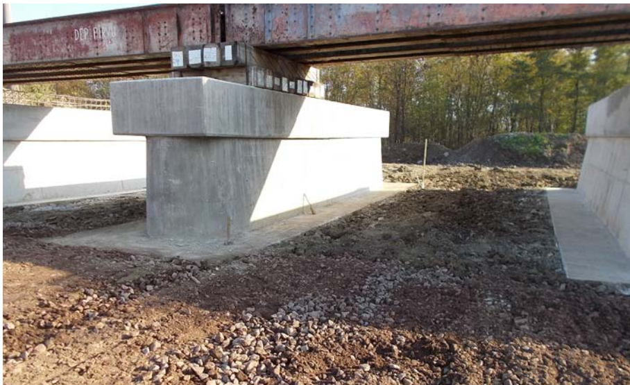
Aspect beton infrastructuri
