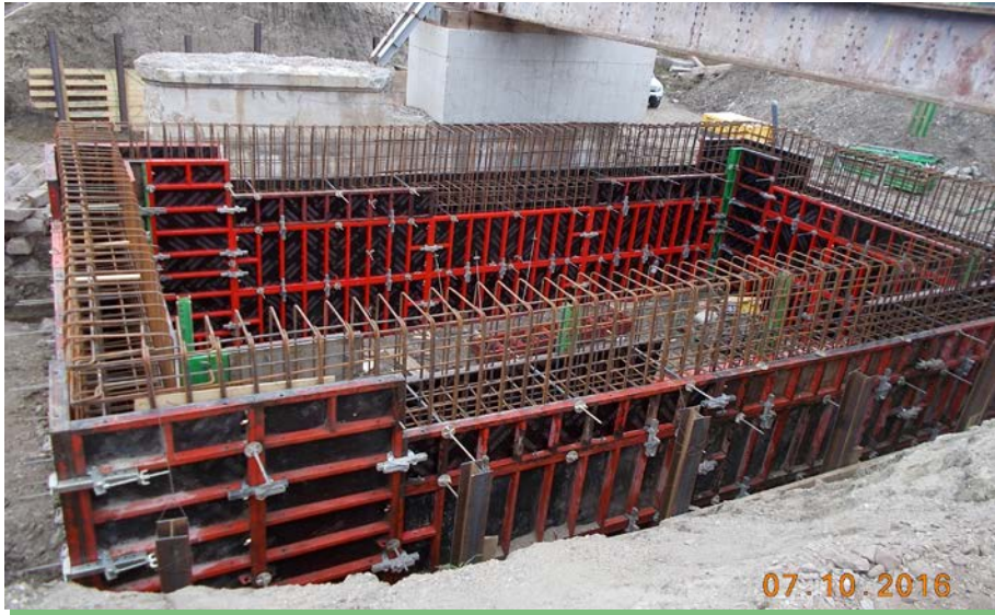
Armare/Cofrare cheson
