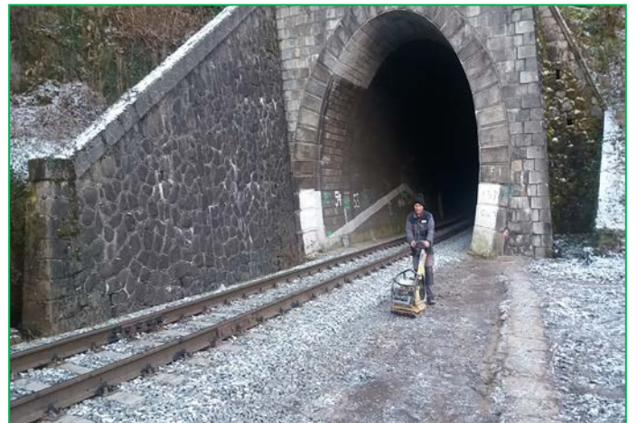
Compactarea banchetei, Tunel Balnaca
