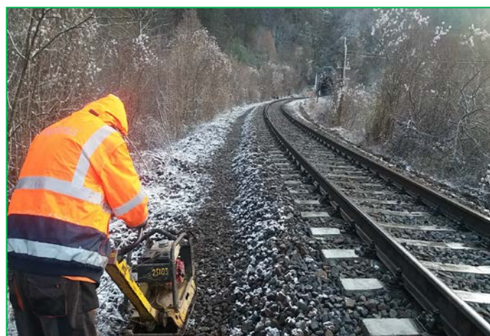
Compactarea banchetei, Tunel Balnaca
