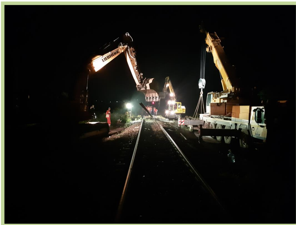
Pod km. 381+660 linia CF Tecuci - Iasi
