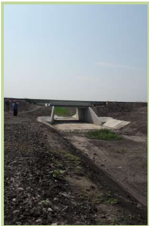
Pod km. 268+678, linia CF Tecuci - Iași
