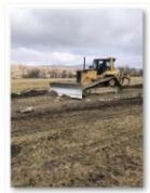
202102-Viaduct km 254+400 - Drum tehnologic_2
