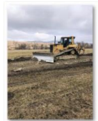
202102-Viaduct km 254+400 - Drum tehnologic_2
