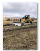
202102-Viaduct km 254+400 - Drum tehnologic 2
