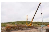
047_executie piloti portal P3 - tunel Homorod
