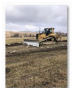
202102-Viaduct km 254+400 - Drum tehnologic_2
