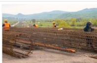
042_executie piloti portal P3 - tunel Homorod
