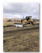
202102-Viaduct km 254+400 – Drum tehnologic_2
