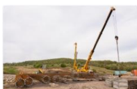
047_executie piloti portal P3 - tunel Homorod
