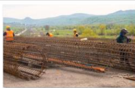
042_executie piloti portal P3 - tunel Homorod
